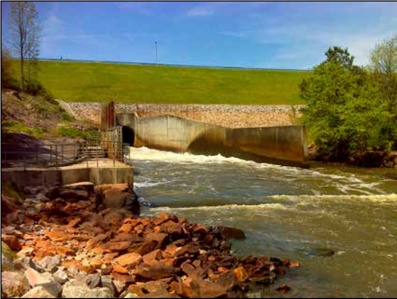
The tailrace at the Falls Lake dam
