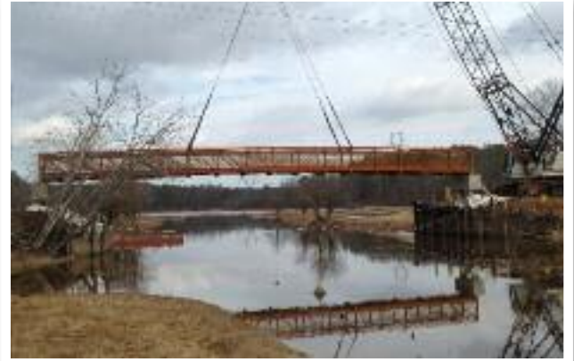
The bridge is installed at Falls Lake. Photo by Gregory Scott
