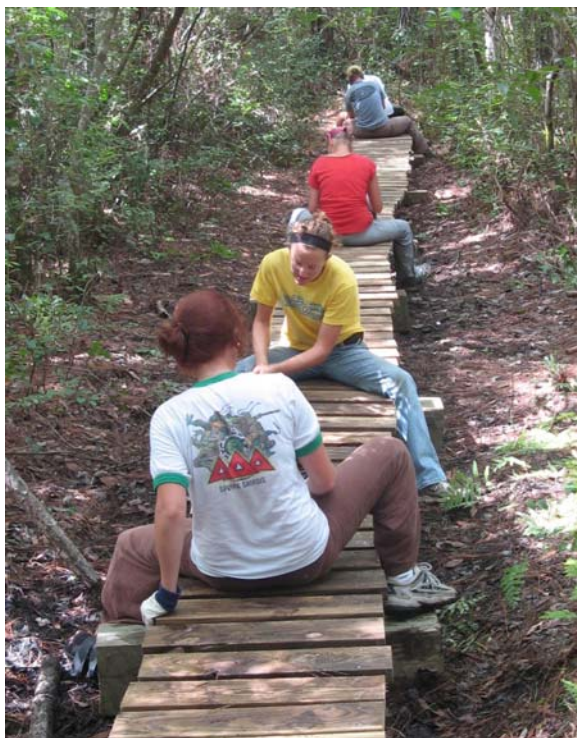
Neusiok Trail/MST – boardwalk construction
